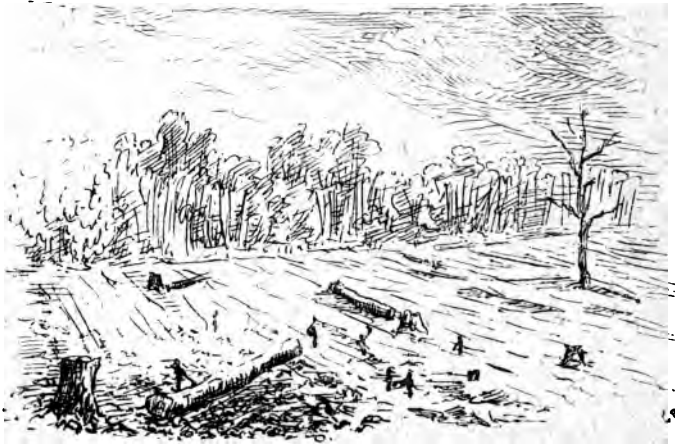
CLEARING THE GROUND.
